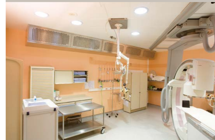
Centre hospitalier Cornouaille, Quimper Cornouaille hospital, Quimper, France
